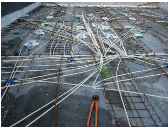
Electricity in ground plate
