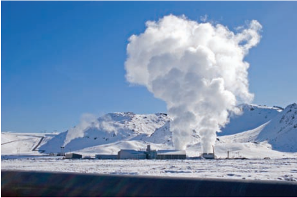
Hellisheiði power plant
